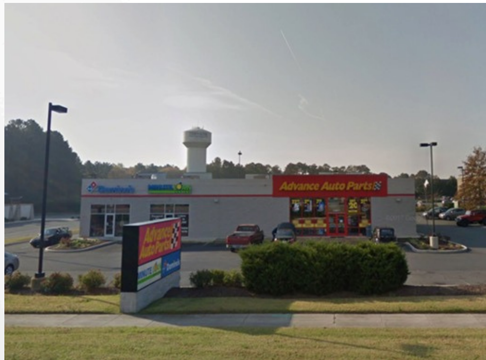
LEWES, DE Advance Auto, Domino's Pizza, Minute Loan New Construction Multi-Tenant NNN
