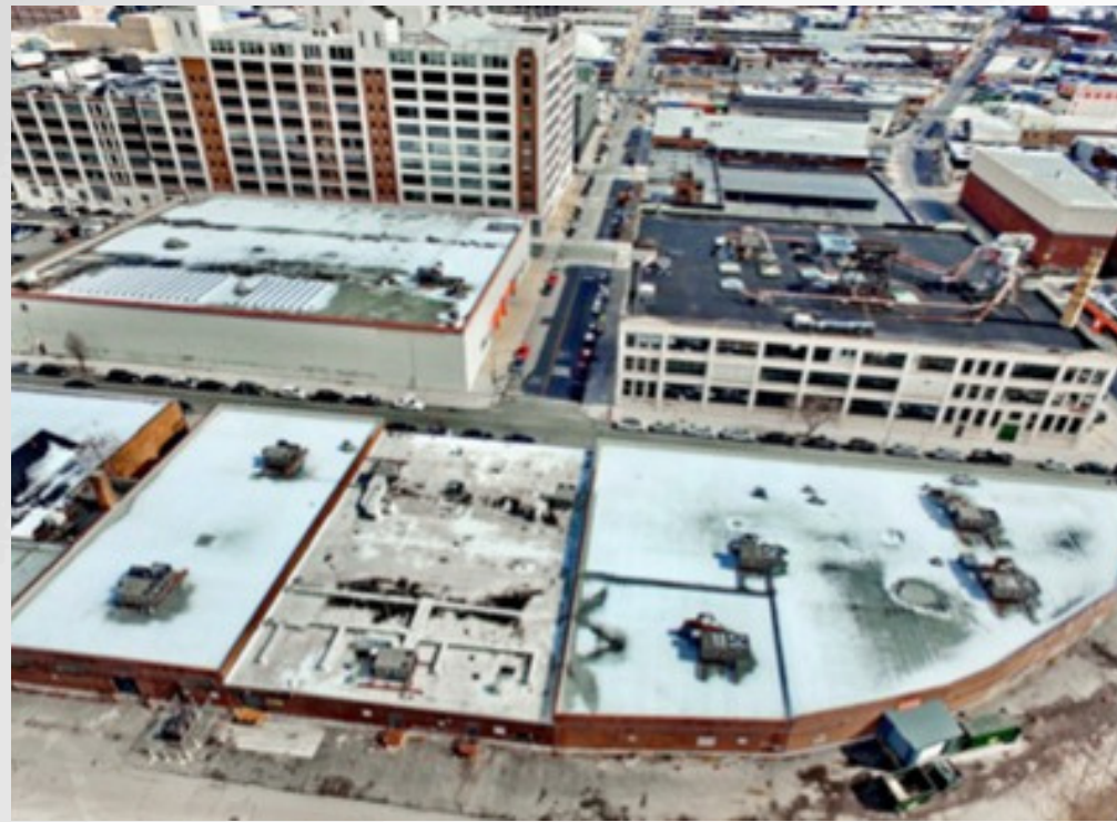
LONG ISLAND CITY, NY 52,000 SF Industrial Property
