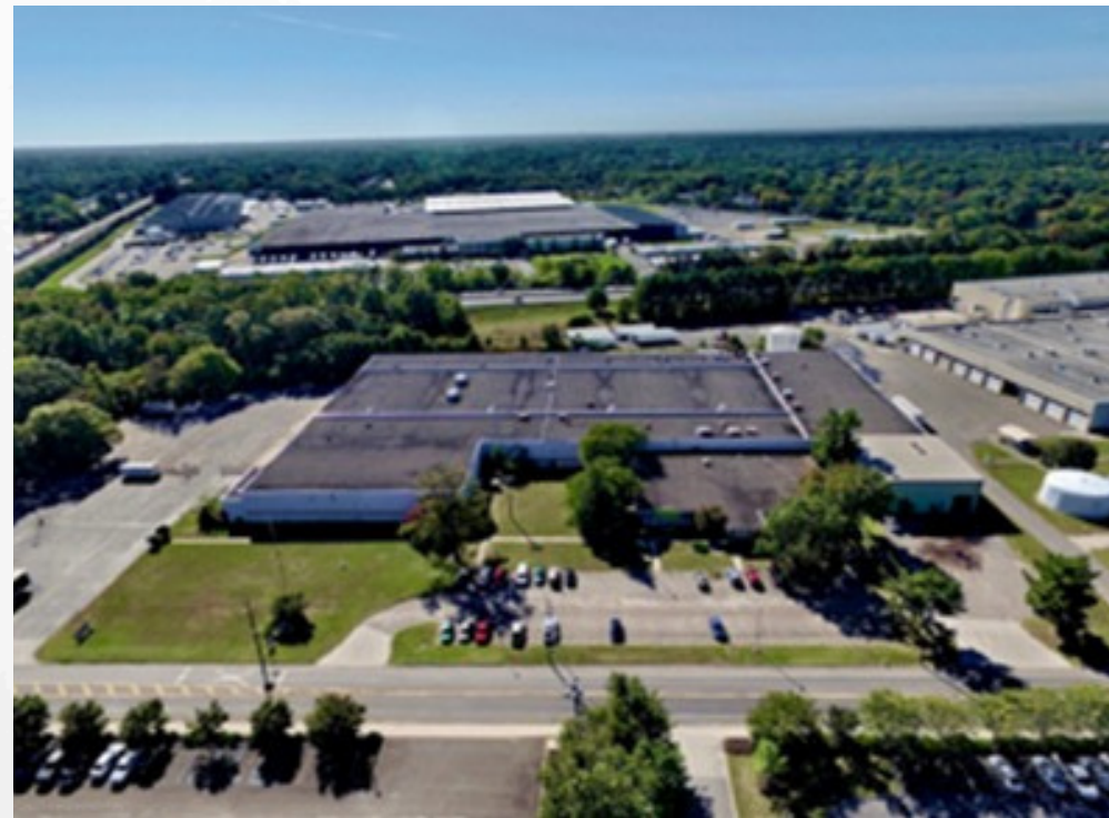
BARRINGTON, NJ 140,000 SF Industrial Property
